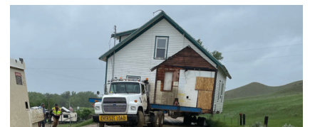
Crew lifting lines for a house
