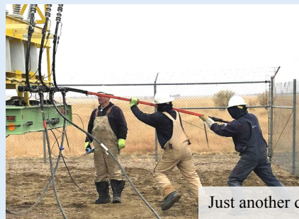
Outback Power, our contractors, work to reconductor the South River Road line in February.
