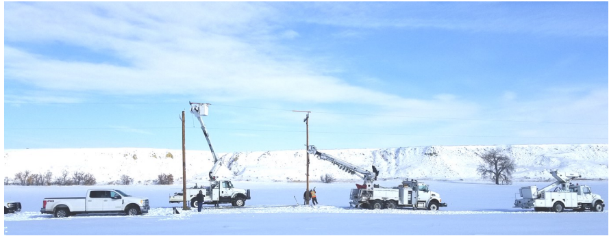
Outback Power, our contractors, work to reconductor the South River Road line in February.
