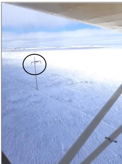
The insulator had burnt off, causing the fault. A fly-over in the daytime made this visible.
